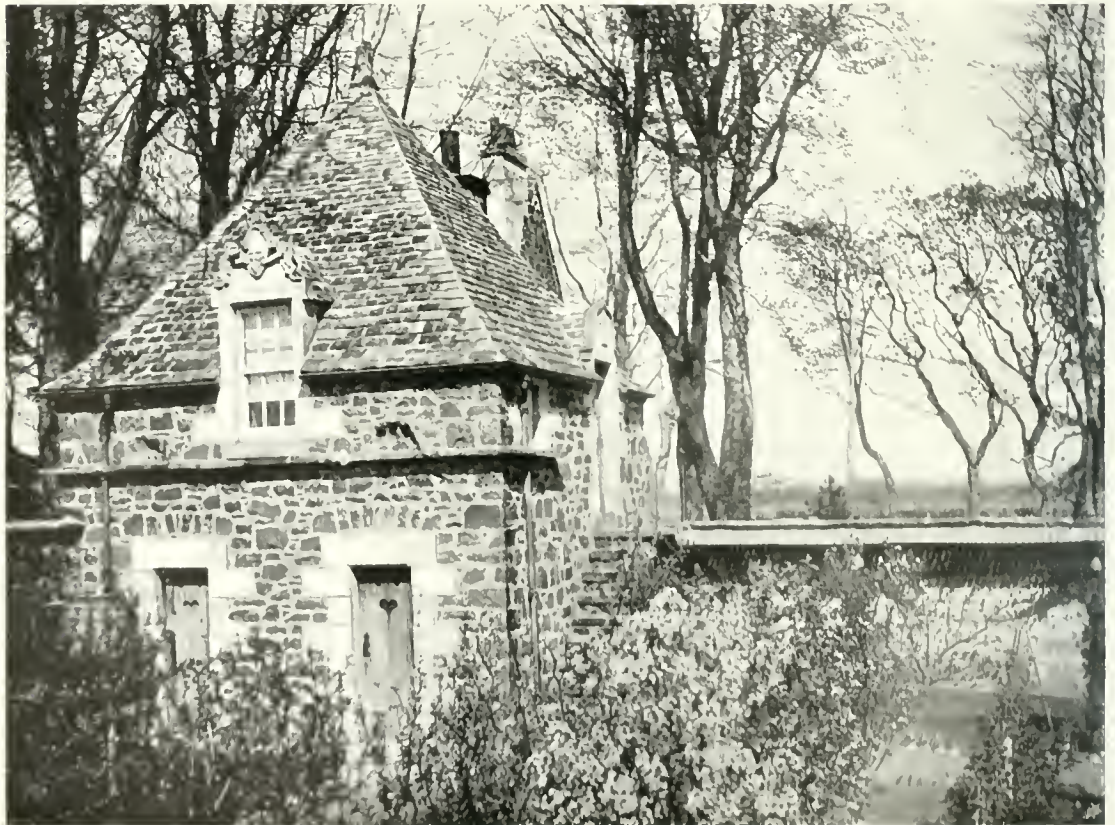
VIEW OF THE GARDEN PAVILION AT FARESHALL, FIFE, BUILT OF LOCAL RUBBLE WORK AND ROOFED WITH ARBROATH PAVEMENT SLATES
